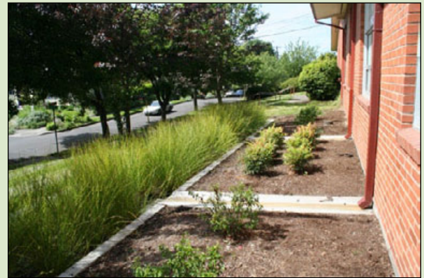
Figure D-7. A flow-through planter adjacent to an apartment complex in Portland, Oregon. This stormwater planter is completely lined to protect the building foundation from migrating water.
