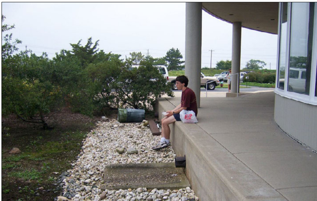
Figure D-2. Downspout disconnection into an infiltration garden at the University of Delaware's Lewes Campus.
