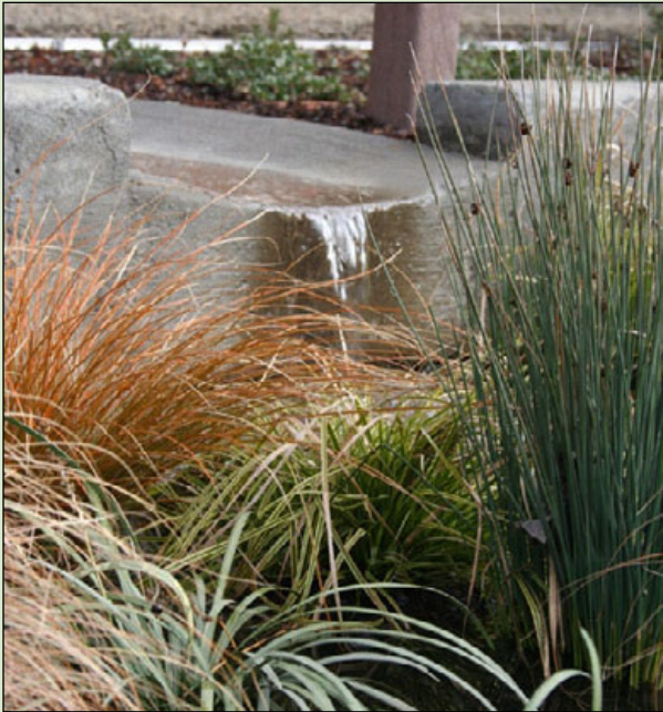
Figure D-9. Water is conveyed on the surface into a stormwater planter via a concrete runnel.
