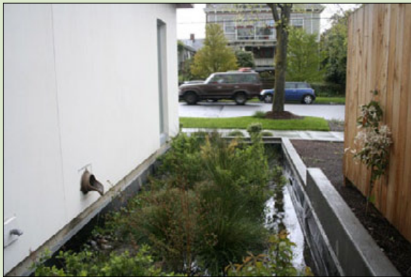
Figure D-6. An infiltration planter located away from the building foundation. Notice the surface conveyance of runoff to the planter by using a concrete runnel.
